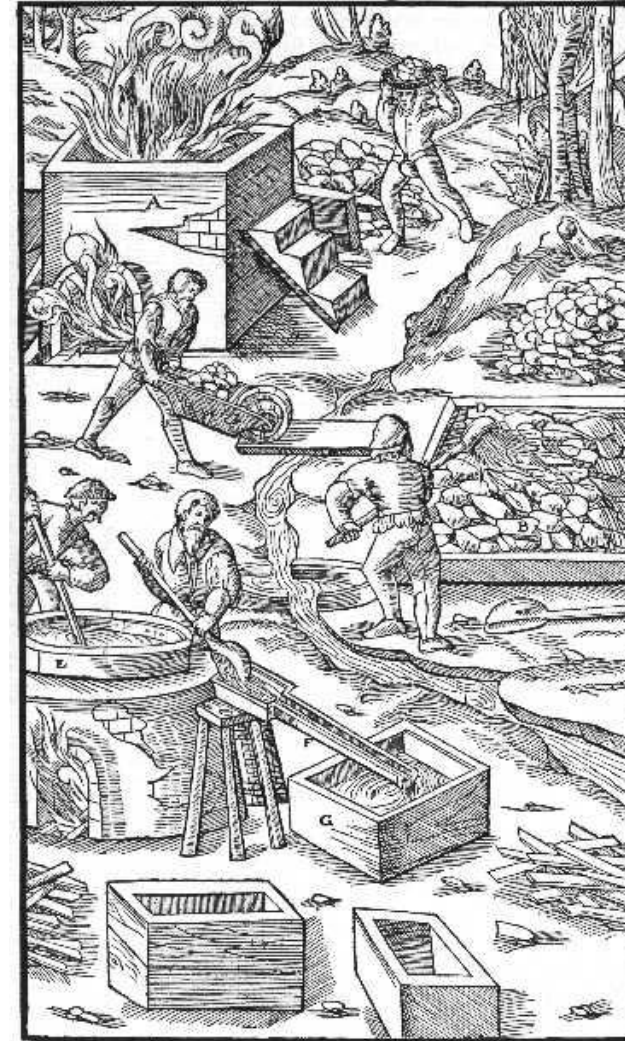
A—FURNACE. B—ENCLOSED SPACE. C—ALUMINOUS ROD. D—DEEP LAIR. E—CALIBRE. F—LAUNDER. G—TROUGH.
